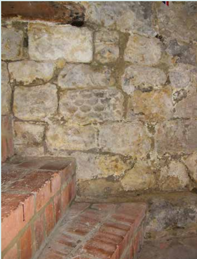
Carvings in cellar of 20 Long Street, Devizes. © Wiltshire Buildings Record
